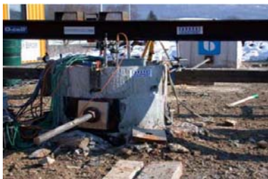
Lateral testing in progress
