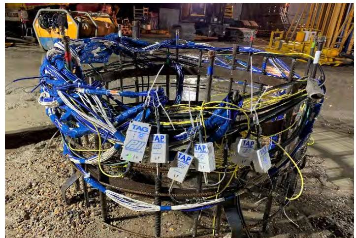
Thermal Integrity Profiling loggers
