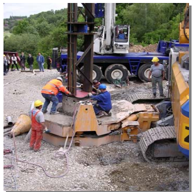
Installation of the O-cells on the steel carrying frame into the pile bore
