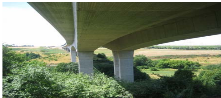
Underside of the completed bridge
