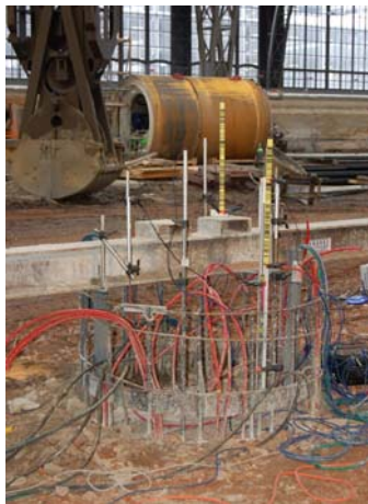
Test in progress (diaphragm wall grab and tunneling machine in the background)
