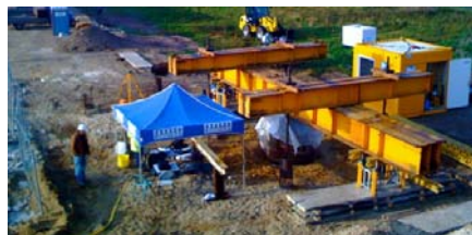
O-cell test alongside a traditional top down assembly
