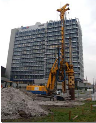
Boring of Test Pile 1 adjacent to existing SWR building
