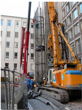
Installation of the bottom section of reinforcing cage with both O-cell arrangements
