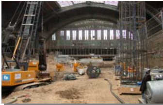
O-cell Assembly Placement
