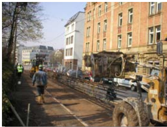
Transportation of the pile cage along narrow street
