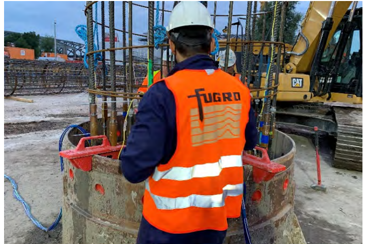
Pile reinforcement installation with O-cell® assembly
